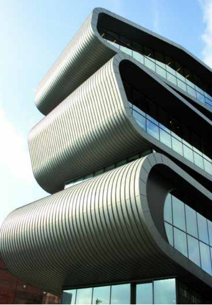
VMZ Dik kenet tonoz kabuk cephe, QUARTZ-ZINC®
